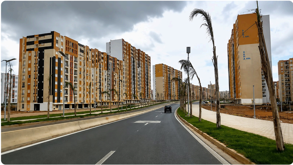
Figure 4: A main boulevard in Sidi Abdellah, the “city of Legos.”
