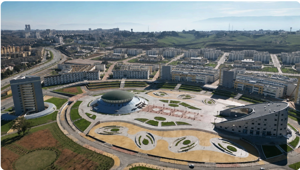
Figure 1: An aerial view of the Sidi Abdellah techno pole.
